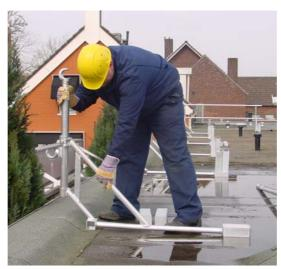
1. Place the frames no more than 3 metres apart. Place the guardrail supports in the highest position in the roof joists with the bottom claw pointing towards the outside of the building. Tighten the connection.
