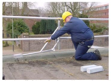
5. The roof joist can be taken off of the roof surface and hung on the support so that material can be passed underneath. To do so, unscrew the connections of the roof joist, slide the roof joist upwards along the frame support, rotate the roof joist a quarter of a turn and tighten the connection by hand. Next, place the roof joist back in the position for use.
