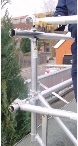
4. Lock the guardrail tubes together using the guardrail securing pins. In the corners of the roof, click the guardrail tubes which are too long into the guardrail connector at the corners of the roof. This guardrail connector is slid onto the guardrail tube and secured in position.
