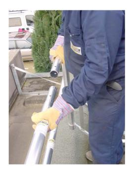
3. Clamp the guardrail tubes at knee and hip height in the claws on the frame supports.
