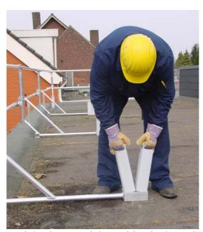
2. Place the two cantilever weights in an upright position in the end of the roof joist (see diagram).
